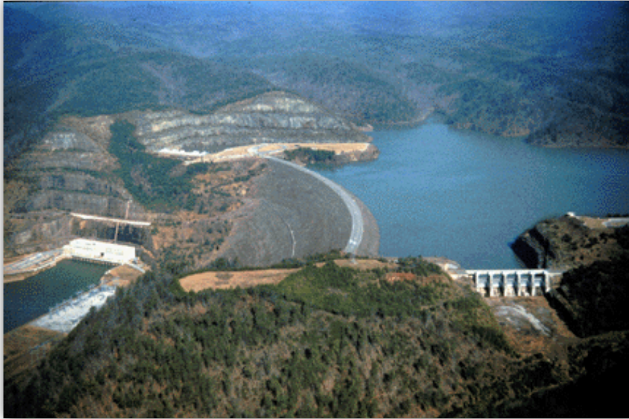
7 8 Figure 2-2 Carters Dam
