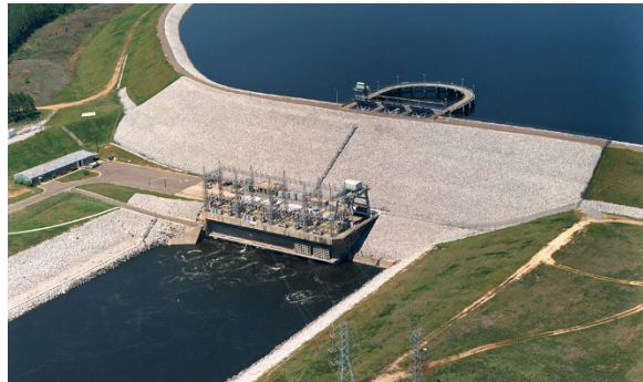
Figure 2-17 Walter Bouldin Dam
